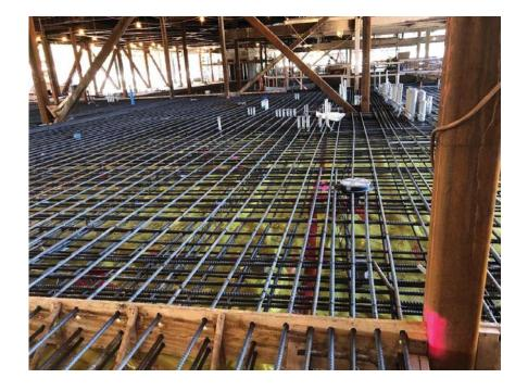
Photo 3 – Auditorium Rebar and Mesh in Place for Upcoming Slab on Deck Pours.
